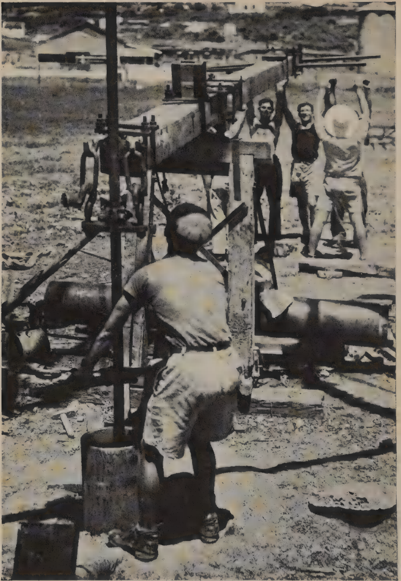
BORING FOR WATER IN A JEWISH COLONY
