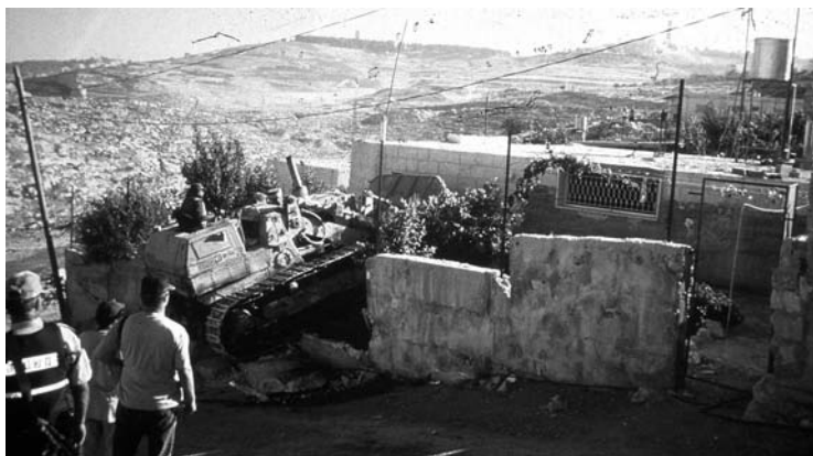
The demolition of the Shawamrehs' home.
